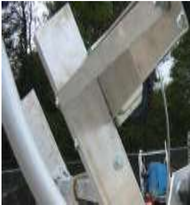
Pontoon arm installation.
