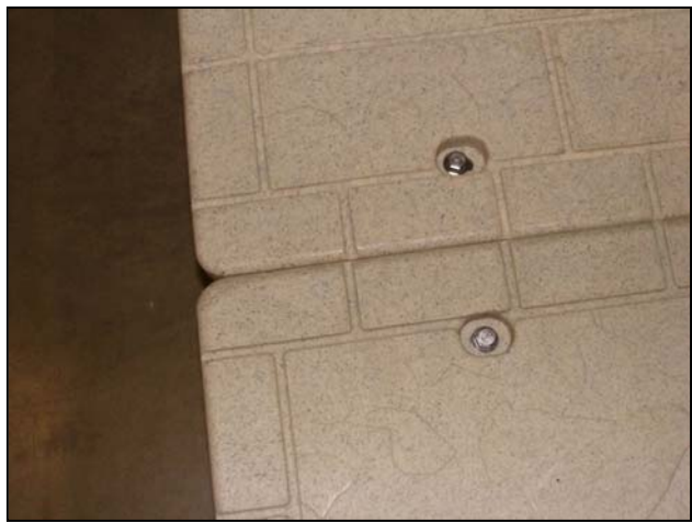
H-Beam Bolted into Dock Sections
