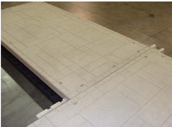
L-Shape with H-Beams sliding into position. H-Beams will not be visible when fully positioned
