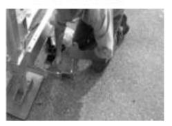
(22) Next, attach the black polypro guide plates in each corner. Insert (5) 3/8"x1 1/2" bolt with washer and 3/8" whiz nut into each hole in the guide plate. You will also need to insert a 3/8"x1 1/2" bolt with a 3/8" whiz nut in the hole on the cradle bracket that the guide plate didn't cover as well as the (3) holes in the bottom inside of the twin beam. The washer is not required for these bolts.
