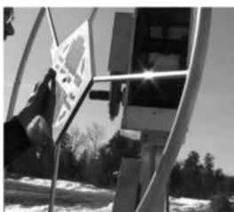
(34) Replace front cover plate on the winch by using a 1/4" bolt on the front bottom and one on the top.
