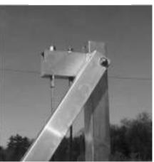
(25) Replace the Winch bottom roller cover plate on the winch with 1/4" bolts. Make sure the rollers are positioned closest to the column. The cable coming out of the winch box must be able to move straight up and down. Next pull the cable from the front Twin Beam with the threaded end and insert through the bottom of the winch and up through the hole in the top of the winch. Fasten with a 5/8" washer and a 5/8" lock nut.
