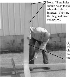
should be on the top when the tube is inserted. They are for the diagonal brace
