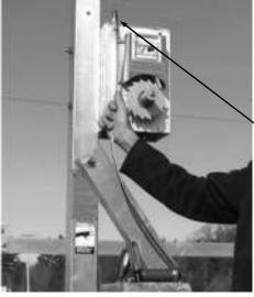
(24) Continue on to the Winch Column Opposite and attach the two cables with the long threaded stud to the welded tube at the top of the column with (2) 5/8" washers and (2) 5/8" nylon lock nuts.
