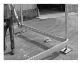
(12) Attach the Diagonal Supports to the Winch Column as well as the Winch Column Opposite. by inserting a 1/2"x 6" bolt, 1/2" washer and a 1/2" nylon lock nut. The Supports are 2"x 3"x 82 1/4" long. Use (4) 3/16"x 3"x 6" long flat bar (shownhere) with (6) 3/8" x 2 3/4" bolts and 3/8" whiz nuts to secure bottom of brace to the Lower Side Panel. Make sure the bolts stick toward the outside of the hoist. This will help prevent any scratching when loading and unloading your boat.
