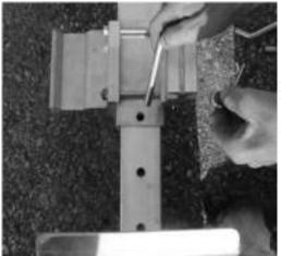
(5) Insert the 7/16" leg pin into the 3rd hole up (approx). This will give you room to work under the clamps. You can adjust after hoist is complete if necessary.
