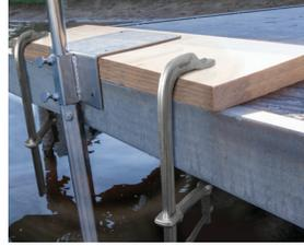
For repositionable installation along longer docks, consider fastening dock mounting bracket to a 2" x 10" x 24" board and securing to dock with sturdy C-clamps.
