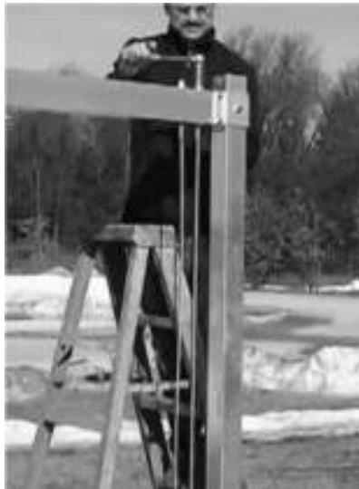
**(24)** Continue on to the Winch Column Opposite and attach the two cables with the long threaded stud to the welded tube at the top of the column with (2) 5/8" washers and (2) 5/8" nylon lock nuts.
