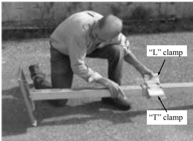
(4) Starting with the Winch Column (96" long) insert the Leg/Foot Pad assembly into the Column. Assemble all four corners the same way. Note: each Column will have a "T" and "L" clamp already bolted to them.
