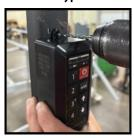
Rotate the keypad assembly out of the way and use a drill and bit to drill a new hole.
