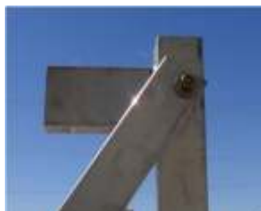
Diagonal Support Connection View on Winch Column Opposite
