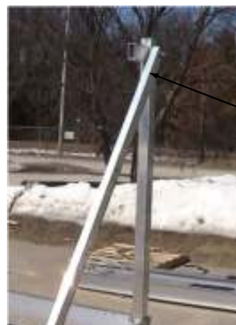
Diagonal Support Connection on Winch Column Opposite
