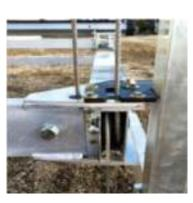
View of cable connection to welded bracket
